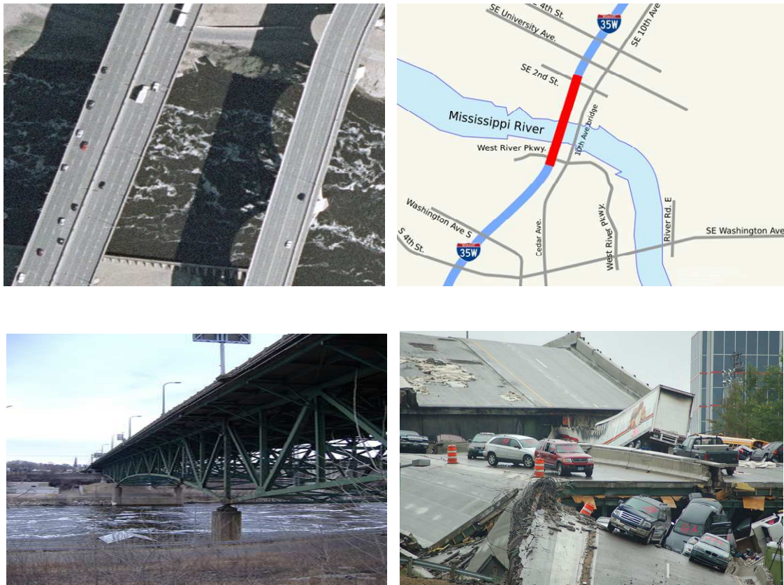
Figure 1.1. Interstate highway bridge I-35W, Minneapolis, Minnesota, collapsed at 6:05 p.m. on August 1, 2007(wikipedia.com).
